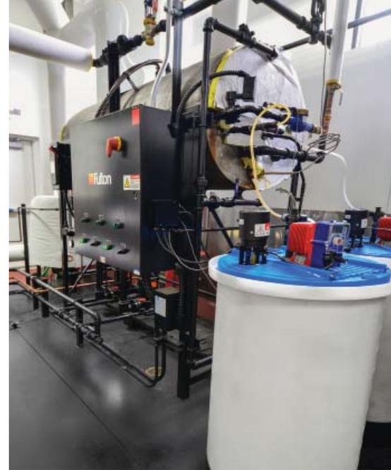
▲ *Fulton skids feature water treatment tanks and a control panel for a condensate return tank to help maintain peak boiler efficiency and culinary steam quality.*
